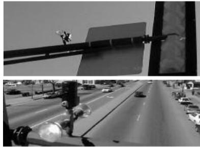
Figure 1. Acoustic Sensors installed at a Traffic Intersection.
